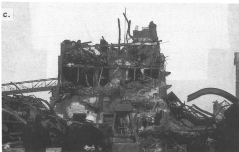
Fig. 1. Pictures of industrial explosion damage. (a) Pernis, The Netherlands, 1968, VCE of hydrocarbons from slops tank, roughly 40 ton TNT eq., (b) Crescent City, USA 1970, BLEVE of propane tank cars, and (c) dust explosion Roland-Mühle, Bremen, 1979.
